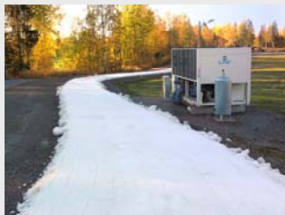
Högbo Bruk Pay & Ski - Placing of underground piping and installation of one of the four chillers. (Photos by ScanRef-Olle Dahlberg)
