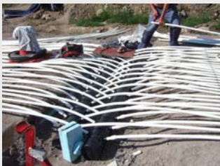
Högbo Bruk Pay & Ski - Placing of underground piping and installation of one of the four chillers. (Photos by ScanRef-Olle Dahlberg)
